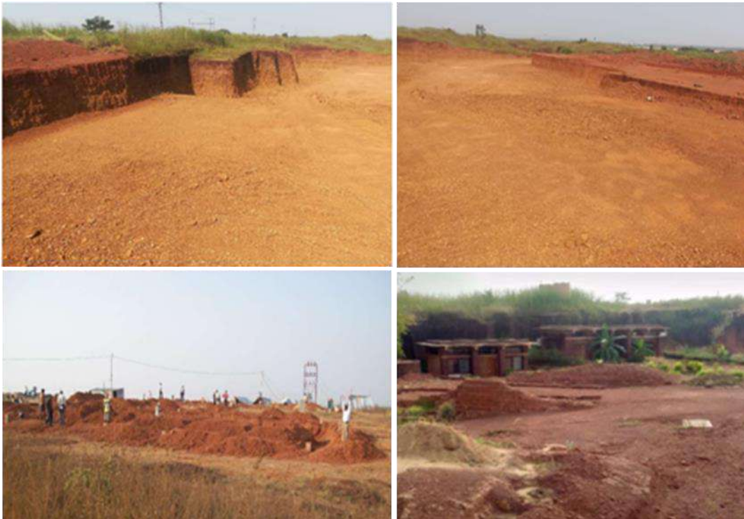
Figure 47: Vast quarry land before the beginning of construction work
