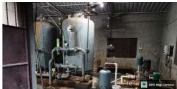
Fig. 4. Drinking water treatment plant
