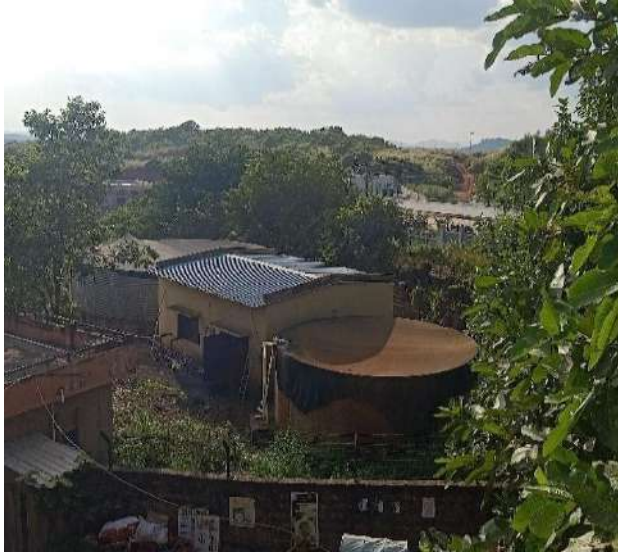
Plate 5. Aerial view of WTP in SSU
