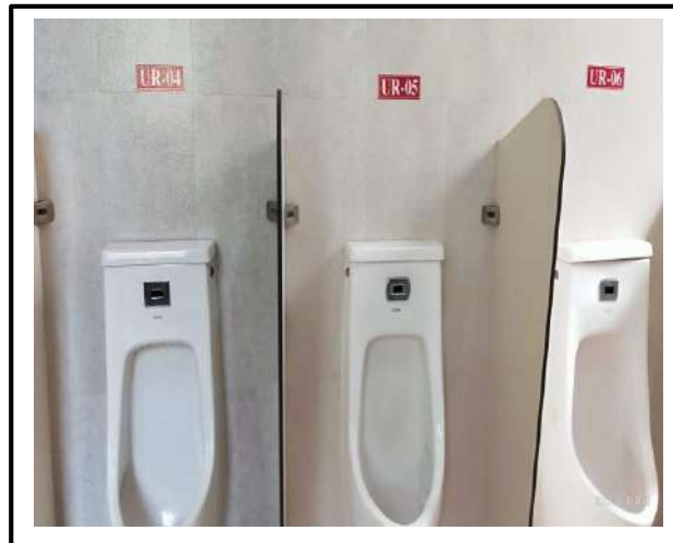
Plate 7.2.2.g Sensor based urinary system
