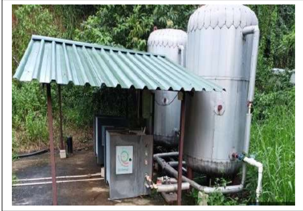
Plate 7.2.4.f. Air sourced water heater
