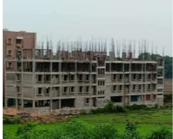
Plate 6. Use of fly ash bricks in the Construction
