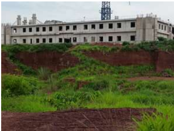
Plate 3. Infrastructure development in a quarry
