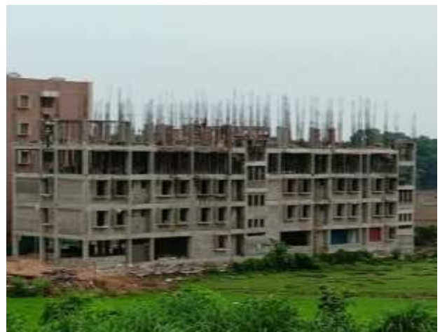
Plate 4. Fly ash bricks for the construction
