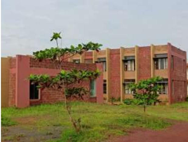
Plate 5. Use of laterite stones in the buildings Plate 6. Construction of playground in a quarry site
