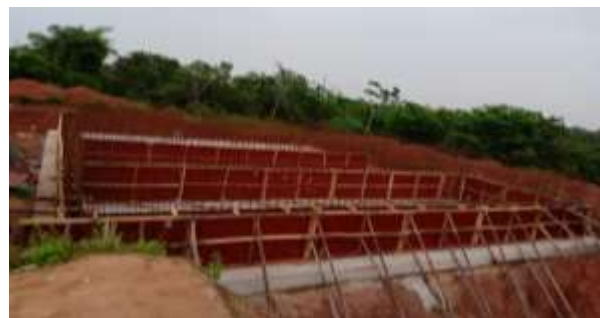
Plate 4. Sewage Treatment Plant under construction
