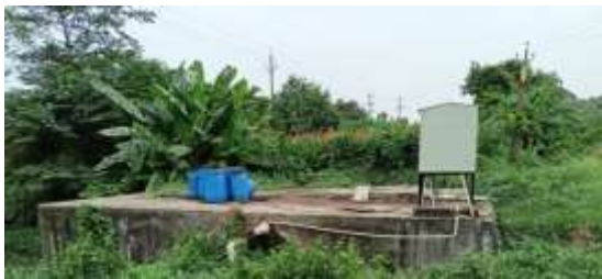
Plate 3. Sewage Treatment Plant
