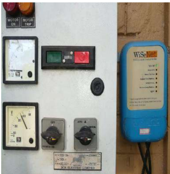
Plate 5. Water level controller in SSU
