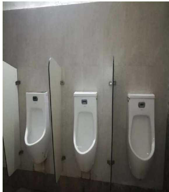
Plate 2. Sensor based urinals in SSU
