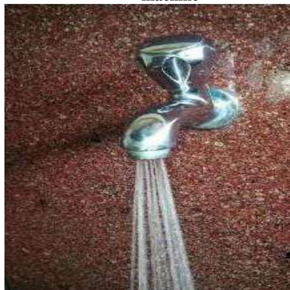
Plate 6. Aerators with faucets
