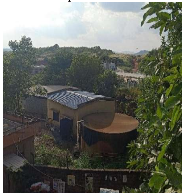
Plate 3. Aerial view of WTP in SSU
