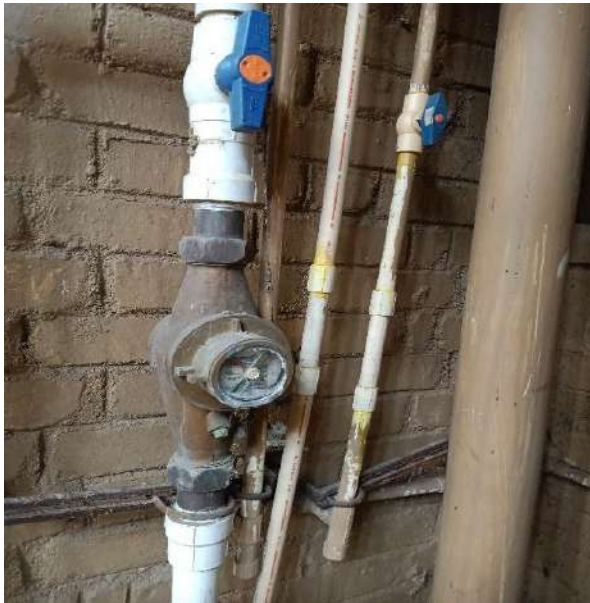
Plate 1. Water meters to track consumption in SSU
