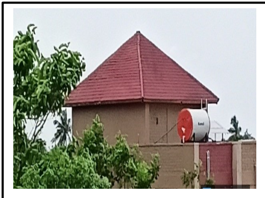
Plate 9 Solar Water Heater
