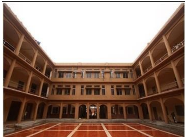
Plate 2. Natural ventilation, lighting and natural laterite stone for construction
