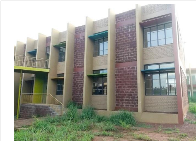
Plate1 .Academic building 'Kirti' is designed for reduced heat absorption and temperature control
