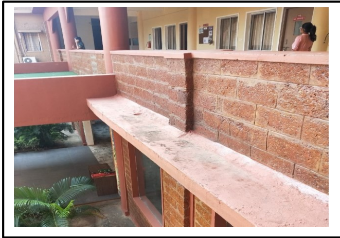
Plate 7 laterite stone building
