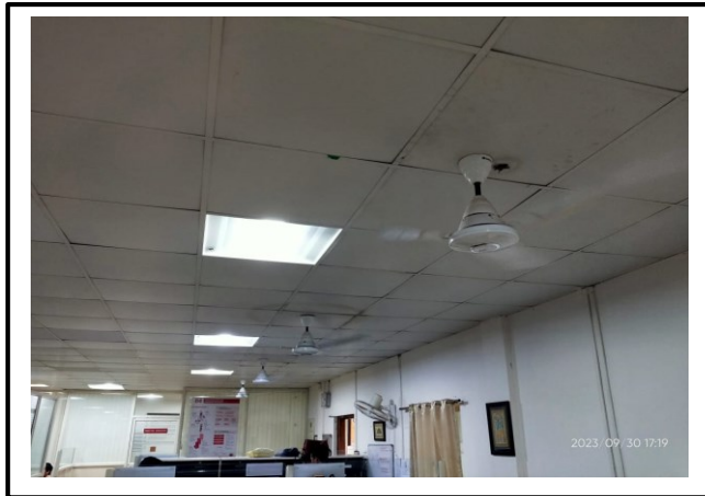
Plate 7.2.2. e. All CFL lamp replaced with LED bulb.
