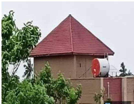
Plate 3. Solar Water Heater at rooftop
