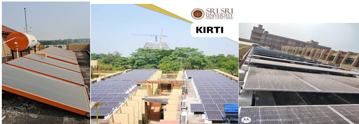
Plate 1. Air sourced water heater and solar plant installation on the roofs of academic buildings
