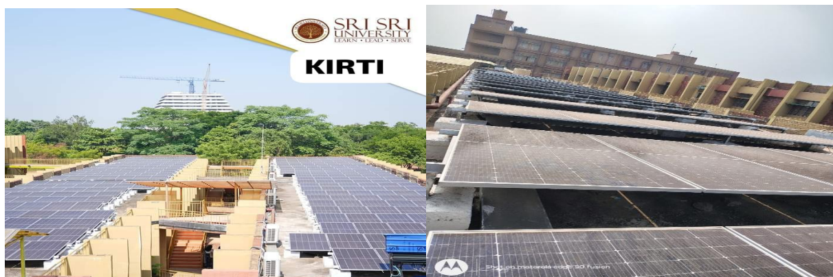
Plate 4. Installation of 2,998 kWh capacity generation solar panels on the campus
