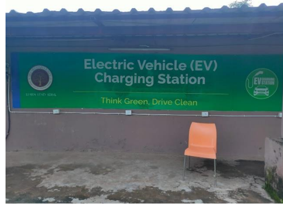
Plate 11 Electric Vehicle Charging Station
