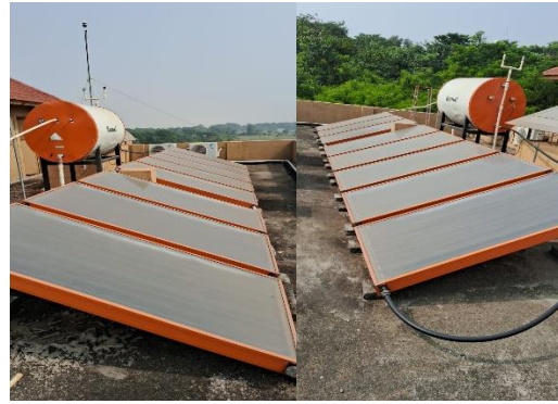
Plate 7.2.4f. Air sourced water heater Machine
